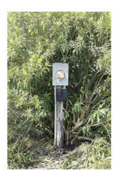
The "new" pier electrical service equipment (above right) recently installed for the pier is very low, even by comparison to other grandfathered non-compliant examples.
