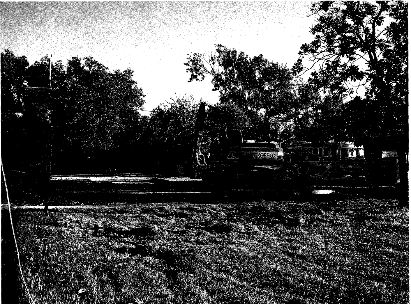
FRONT VIEW OF LOT & DEMOLISHED RESIDENCE
