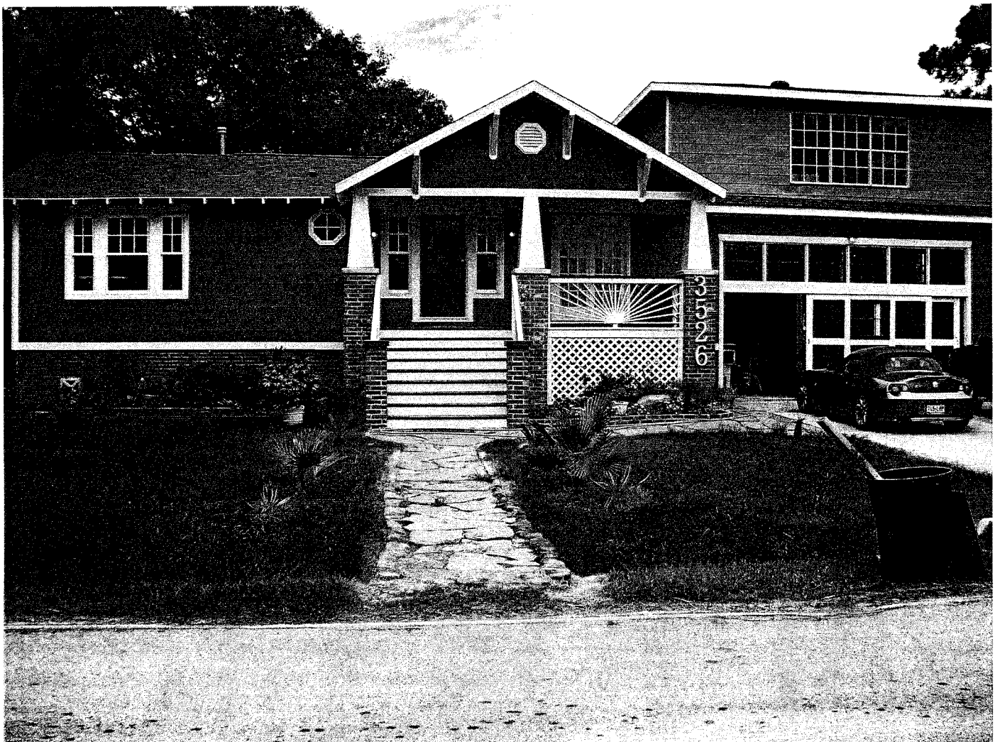
FRONT VIEW OF RESIDENCE W/ATTACHED GARAGE
