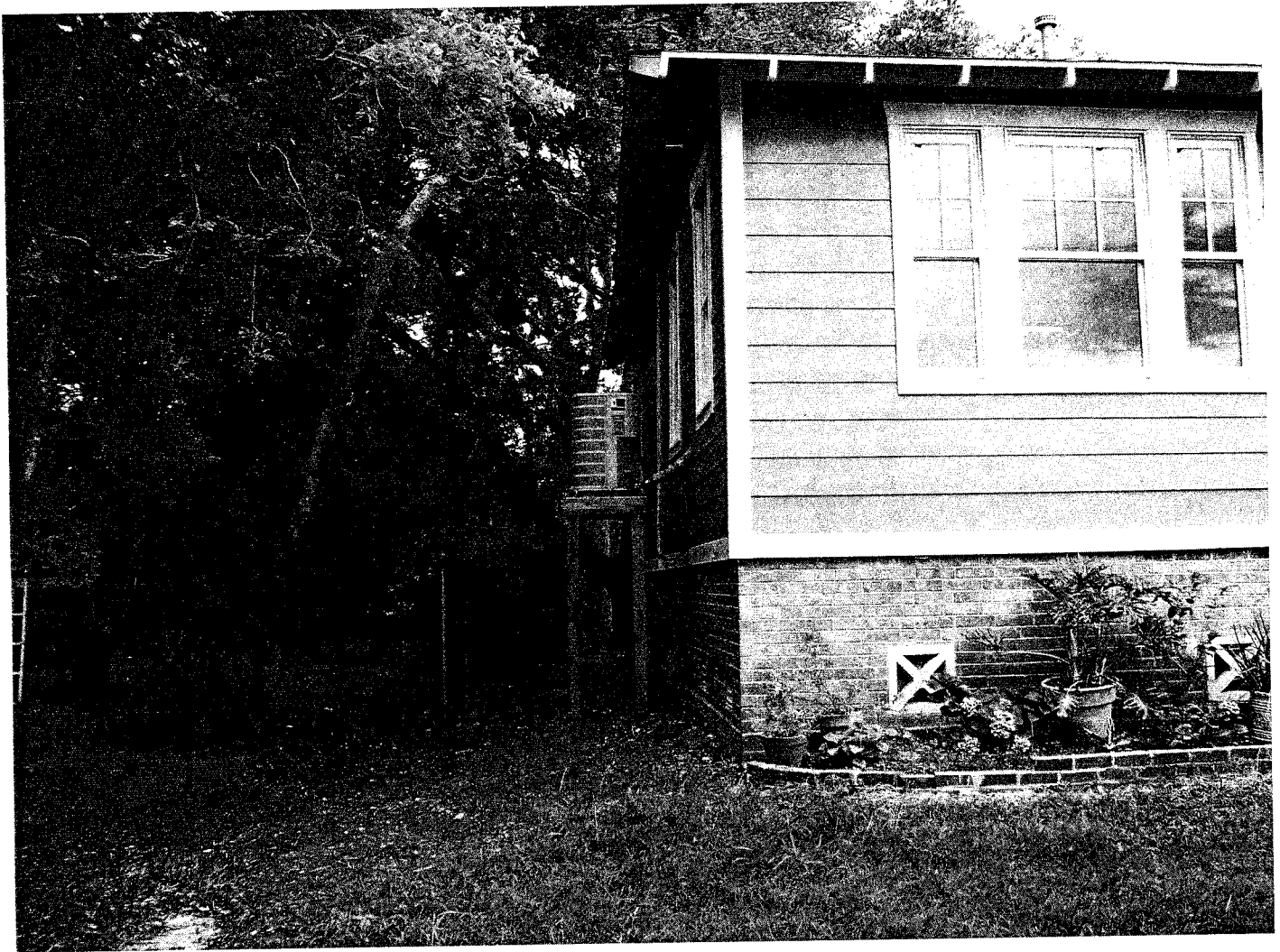
A/C UNIT ON PLATFORM ON SOUTH SIDE OF RESIDENCE
