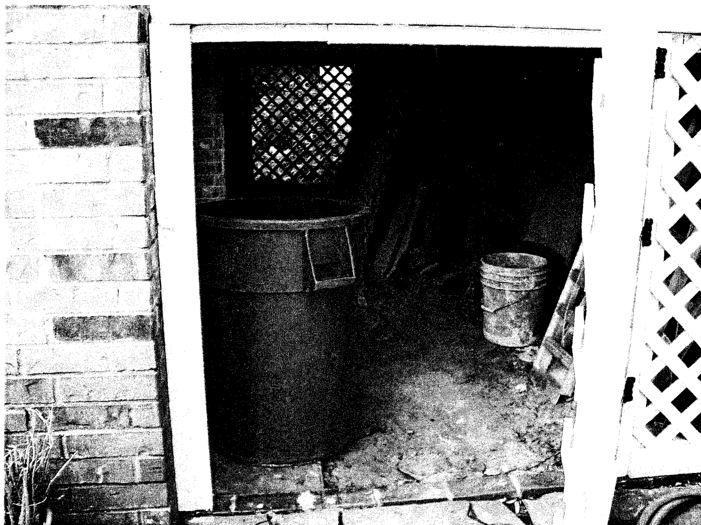
CRAWL SPACE UNDER FRONT PORCH
